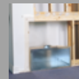
Zero Clearance Box positioned in framework on 50mm Hebel Blocks
