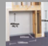
Timber framework, partially clad with 50mm Hebel Blocks
